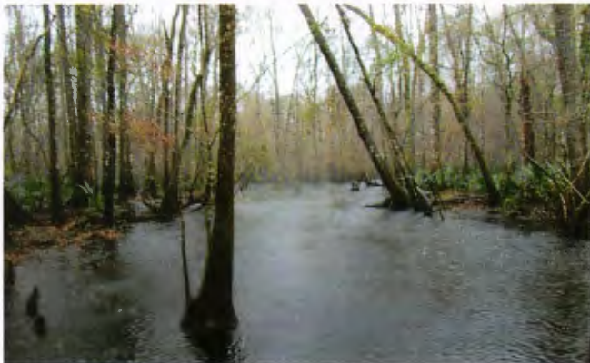
FIGURE 23 Thomas Creek during desnagging process
