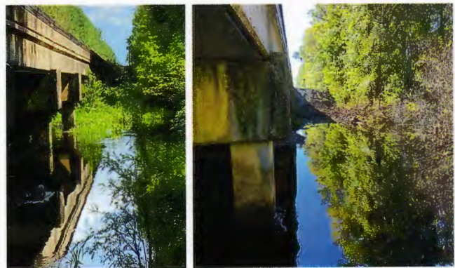
FIGURE 11 (Left) before clearing (right) After clearing CSX Bridge ballast
