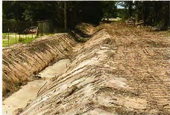
FIGURE 13 New ditch cleared behind Dornbush Rd
